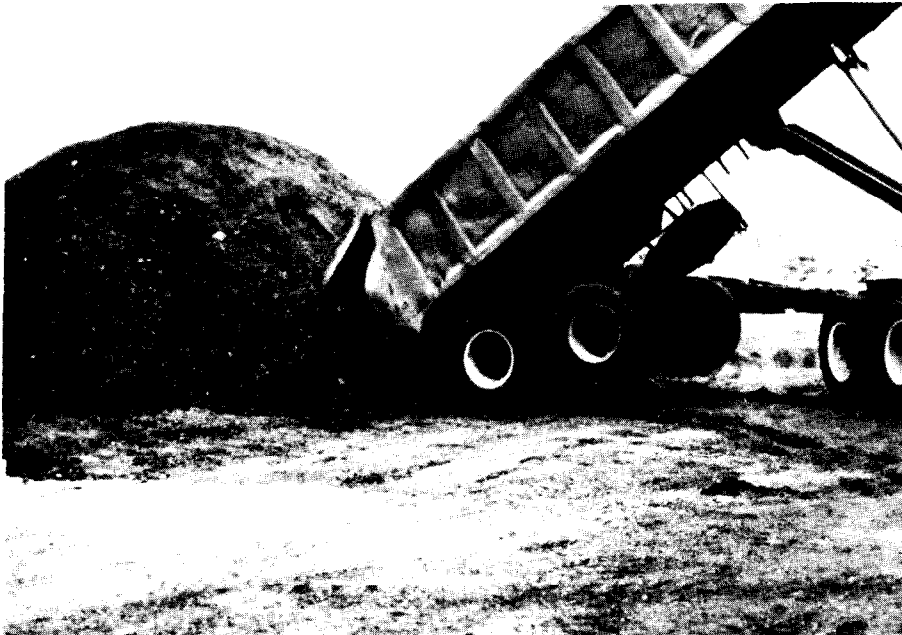
Stockpiling Reclaimed Material
